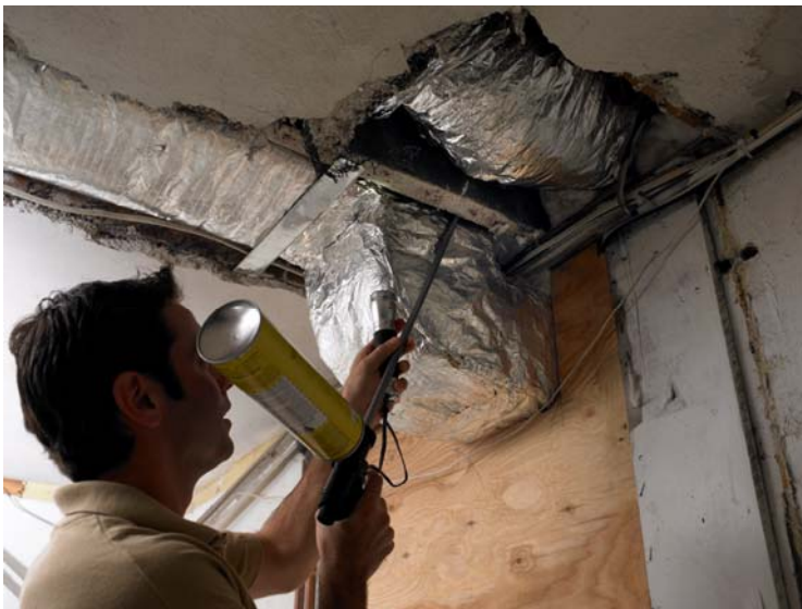
Sealing air leaks by blowing foam into leaky space
